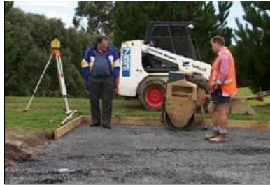
Compacting the base
