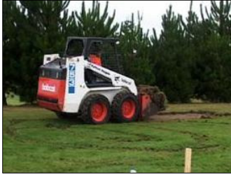
Removing the turf
