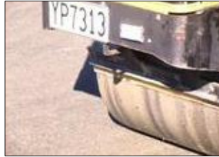
Vibrating roller compacts the crushed lime
