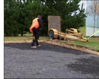
Laying the gravel base
