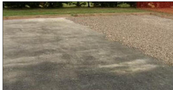
Spreading the top surface over hard base
