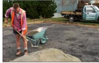
Spreading crushed lime over the base
