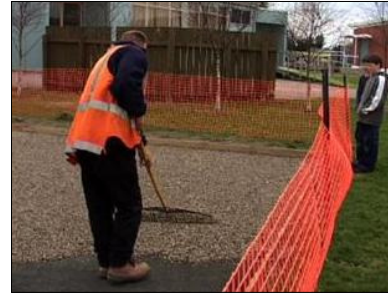
Spreading the top surface over hard base
