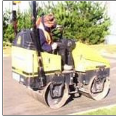
Vibrating roller compacts the crushed lime
